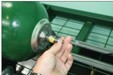
2. Remove the Gas Valve Assembly Cap.
