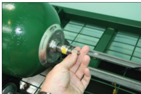
2. Remove the Gas Valve Assembly Cap.
