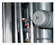
A rotatable display allows the process temperature to be viewed from any angle.
