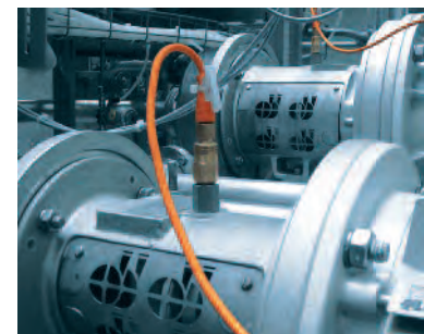
Accelerometers type VSA are connected to VSE units to monitor critical components of the process (pumps, motors, agitators).
